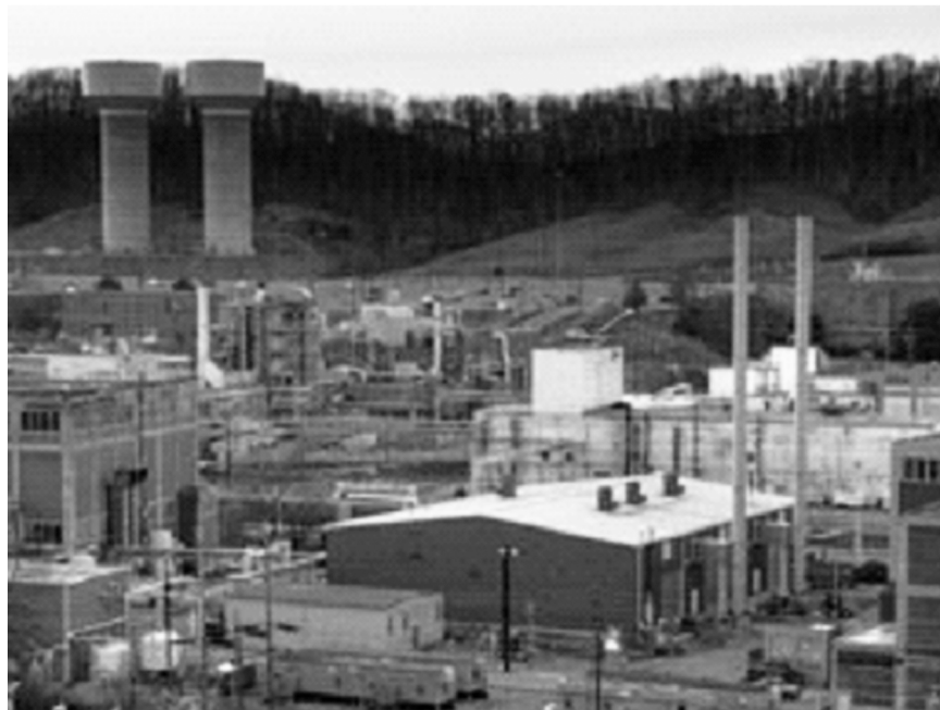
Fig. 4.1. New tanks for the potable water system can be seen in the background, while in the foreground is Y-12's new, natural-gas-fired steam plant.
